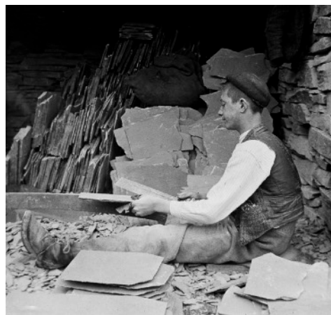
Trimming roofing slates to shape, Langdale slate mine, Westmorland. Photograph taken by Percy Lund circa 1910. ©Clarence O. Becker Archive.
